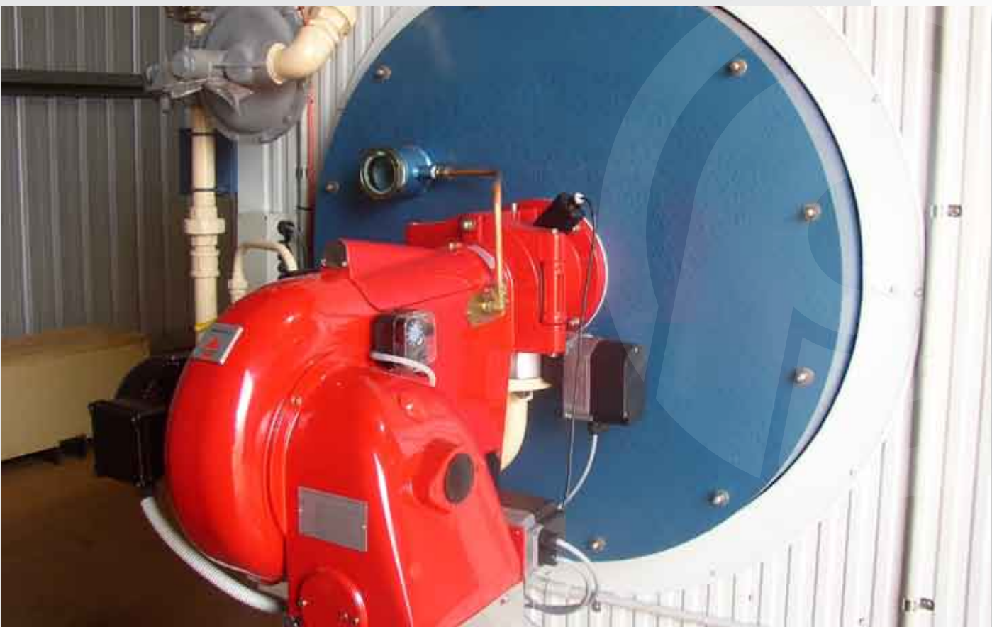
Plenum and Combustion Chamber including 1 000 kW Gas Burner
