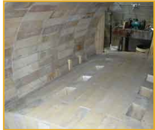
Incinerator Combustion Chamber
