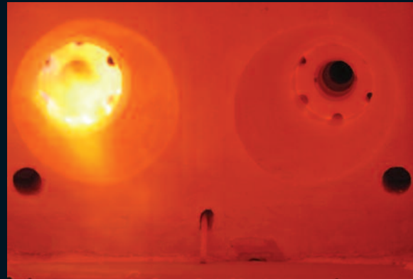
E-Jet Ultra Low NO x Regenerative Burners operating in flameless mode
